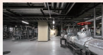
Cold water and steam produced at energy plants are supplied to various facilities through underground piping.
