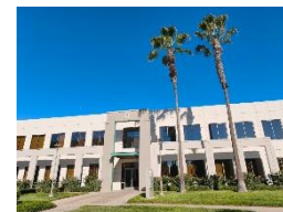
September 2026 KOEI TECMO AMERICA Corporation Opened an office in Los Angeles
